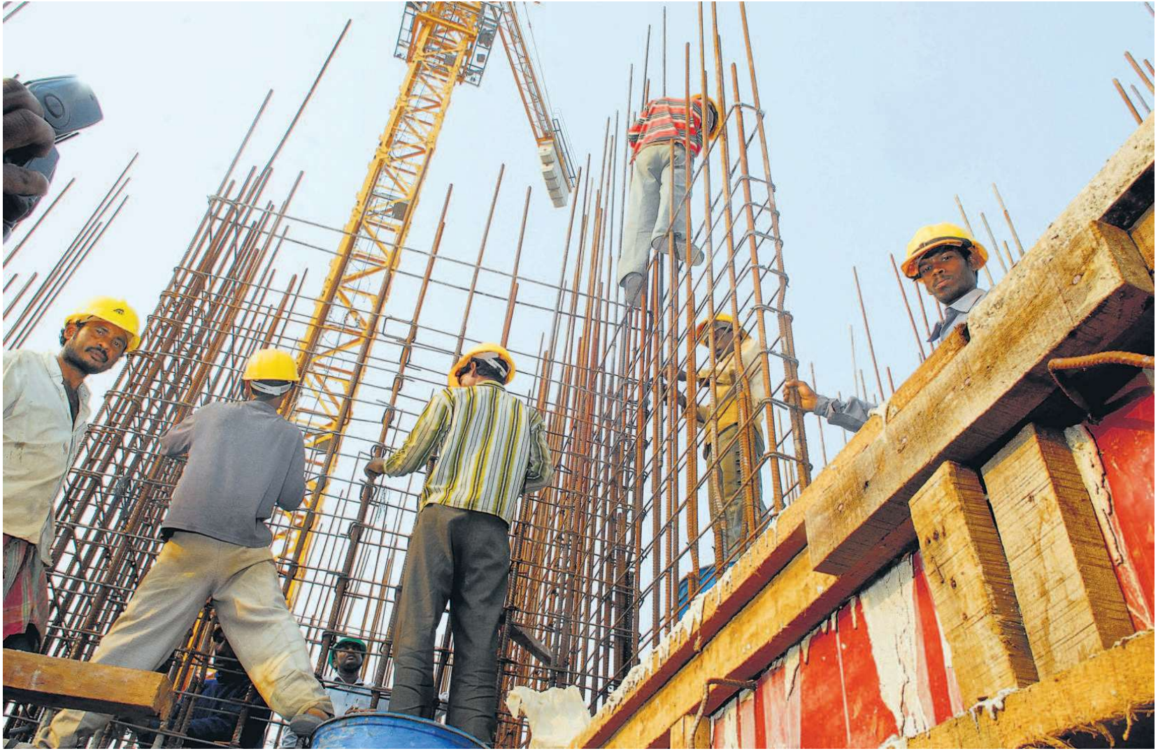
File photo of construction workers at a building site.
